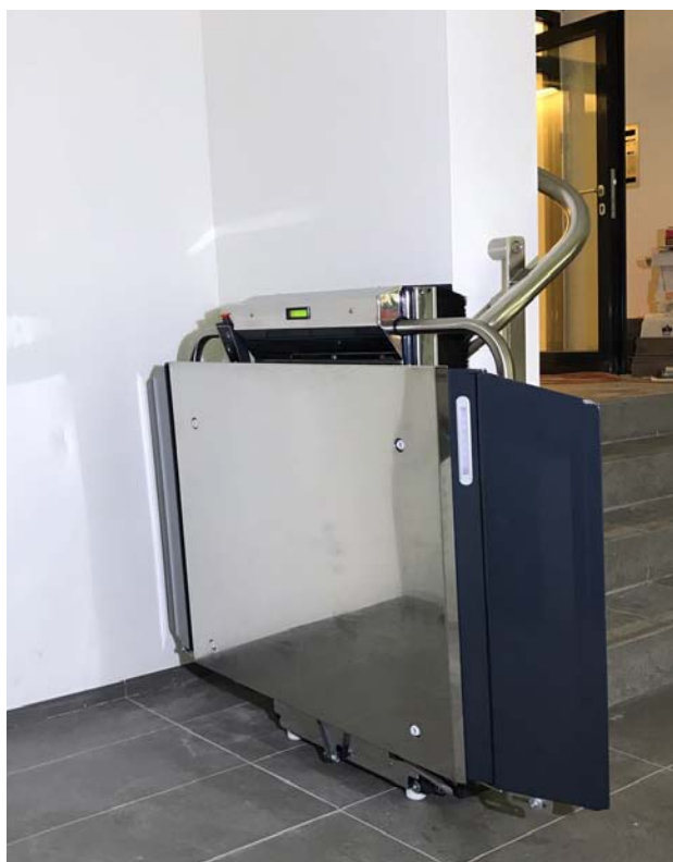
Compact folded platform with metal covers is well secured against vandalism in public spaces
