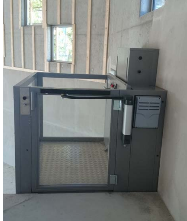
Upper gate with automatic door opener
